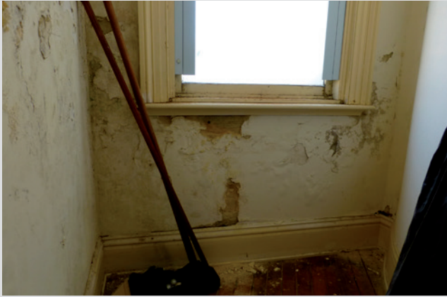
Damage from rising damp on the internal face of wall (above) and external face (below).
