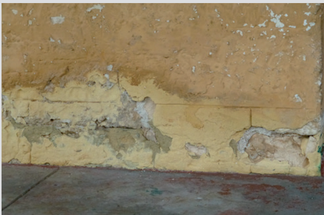
Damage from rising damp on the internal face of wall (above) and external face (below).
