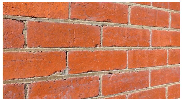
Stretcher bond - Regular courses of stretcher bricks indicate cavity construction brickwork.
